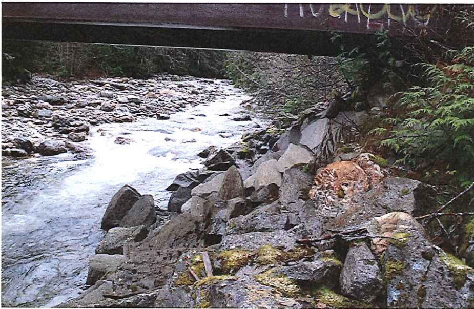
CK2018 Left Abutment
