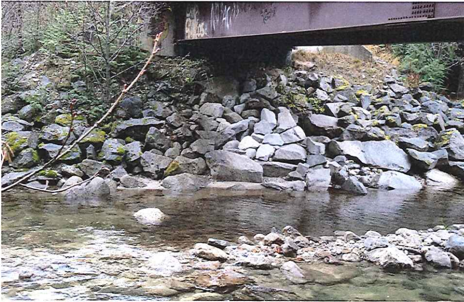
CK2018 Right Abutment
