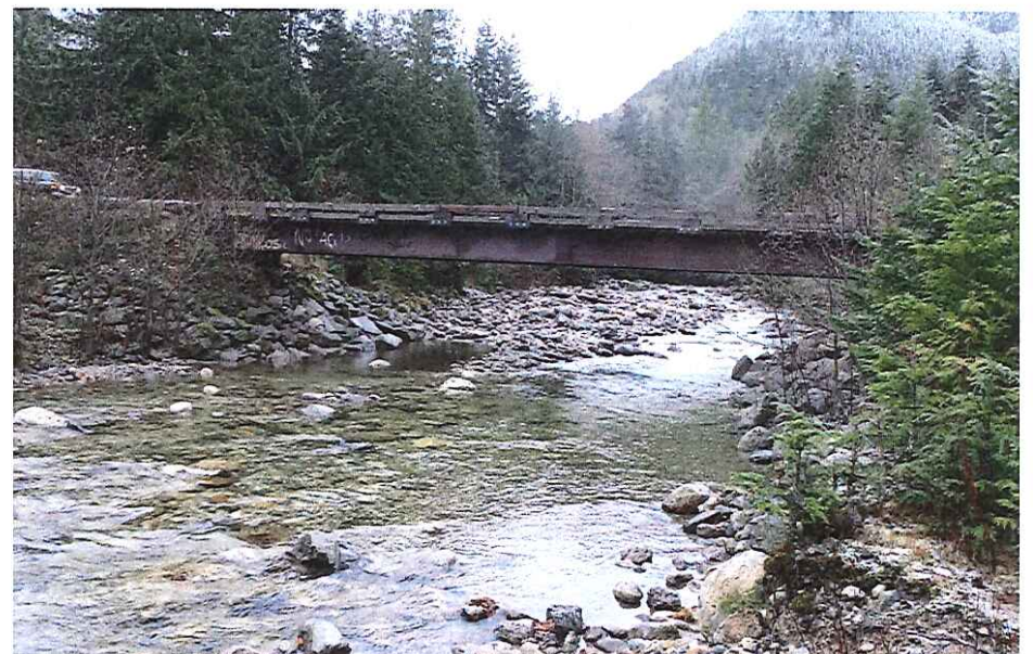
CK2018 From Downstream
