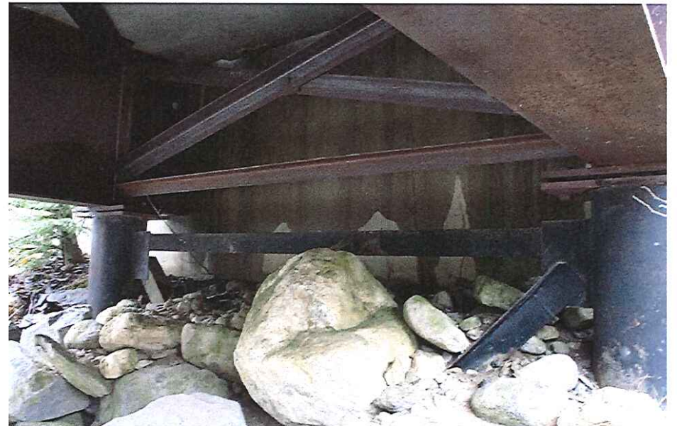
CK2018 Left Abutment Bearing
